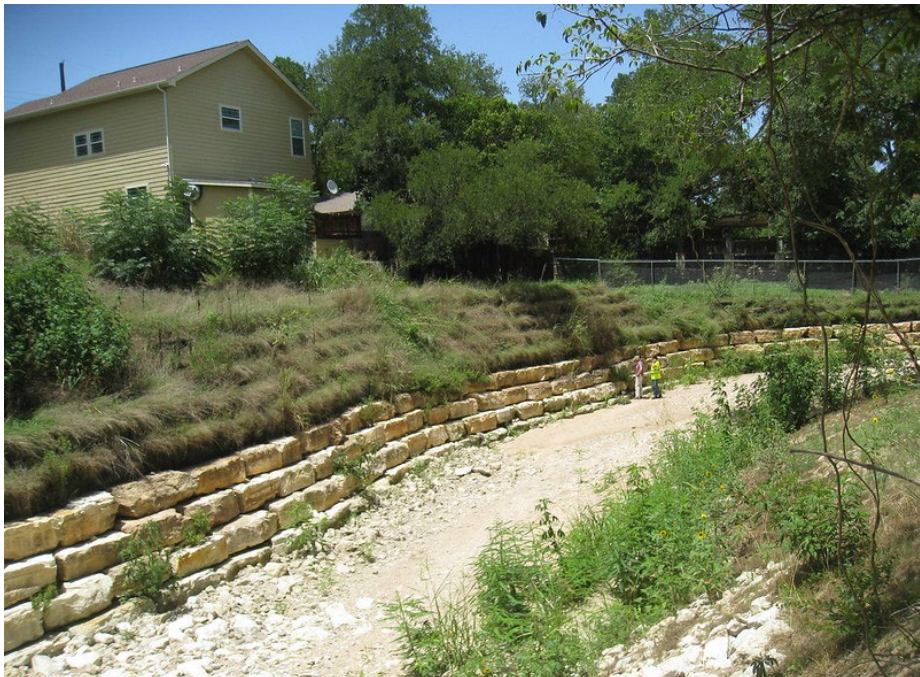
Streambank Stabilization in Austin, TX. Image by City of Austin Watershed Protection
